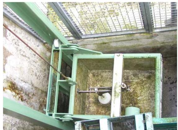
**Figure 6.13. Lift hopper at Ville Hatte Dam eel lift in lower position.**
