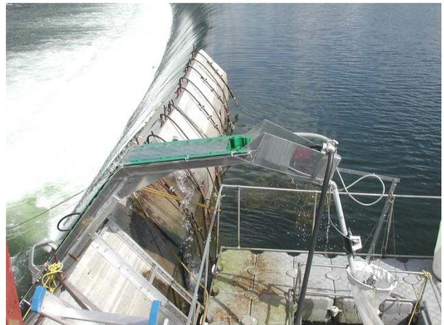
**Figure 6.8. View of Chambly Dam eel pass from above. Note covers over the channel containing the substrate, and the electronic counting device on the pipe carrying the eels from the top of the pass to the keep net. Photo D. Desrochers.**
