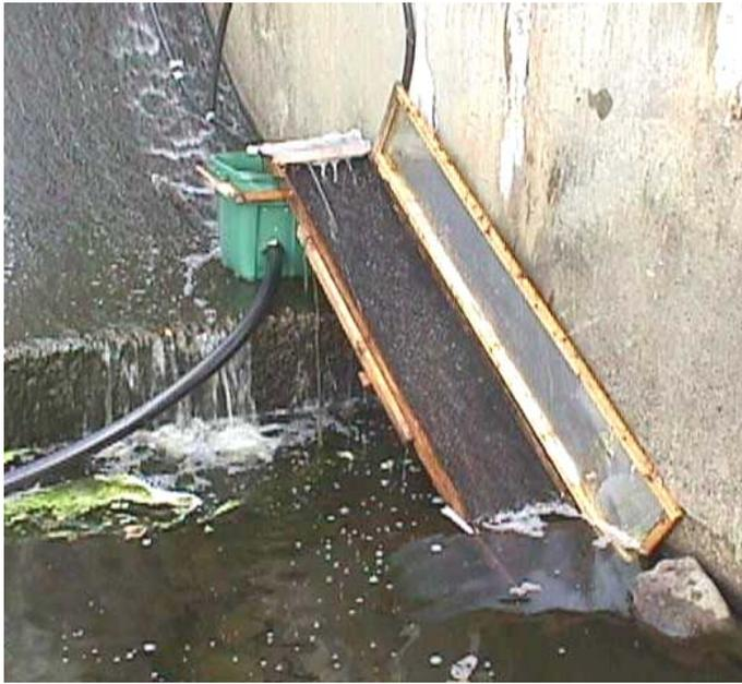
**Figure 6.16.** A “portable passage” being operated at Benton Falls Dam in Maine. The cover is lifted to show the Enkamat substrate. Photograph G. Wippelhauser.
