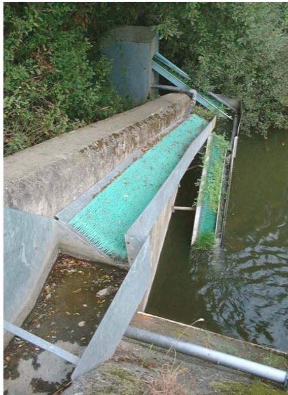
**Figure 6.3. Upstream pass and pass-trap at Pont-es-Omnès**
